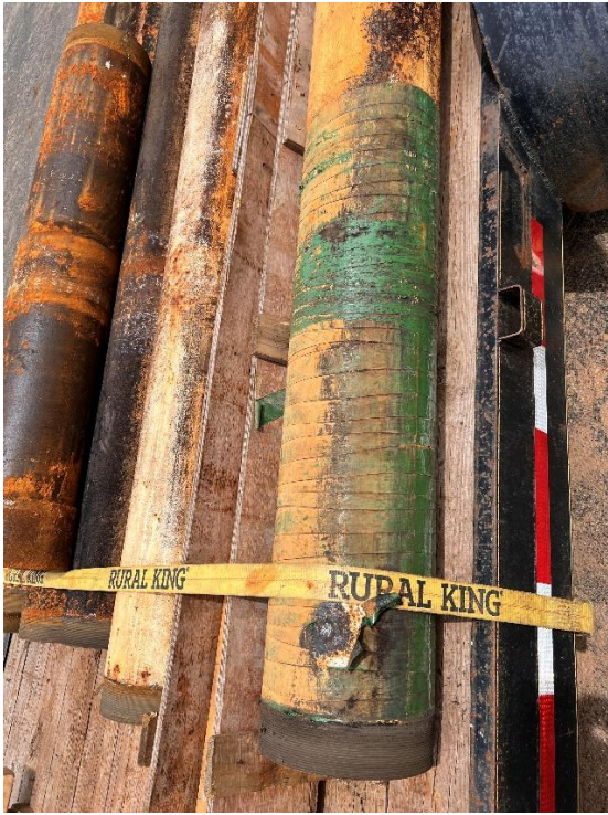
Photo #5: View of Column Pipe Wrapped in Tape. Tape was Covering Large Pits in the Column Pipe. Uncertain Whether Pits Caused by Tape or if Tape Used to Cover.
