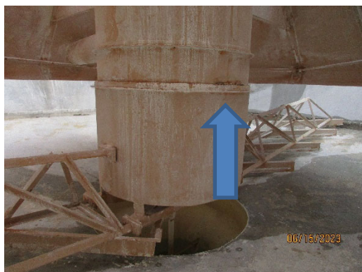
The re-circulation drums are rubbing and need to be aligned or modified.
