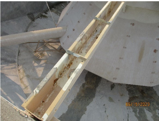
The launders are starting to rust and need to be re-coated. The coatings are peeling off and should be sandblasted and re-coated.
