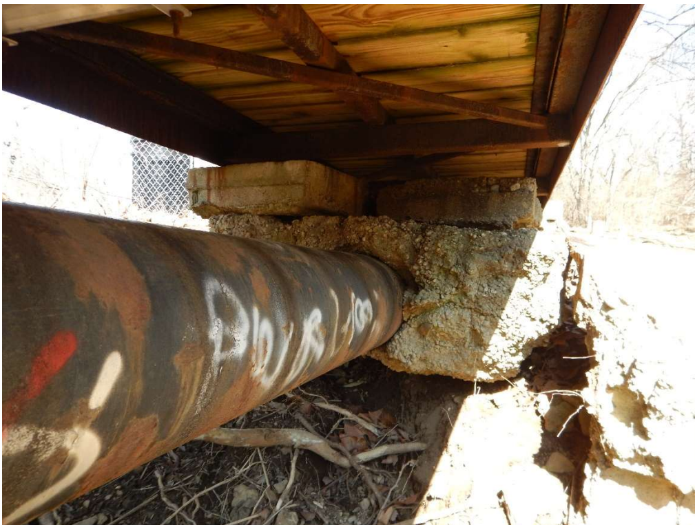
Utility Conduit at North End
