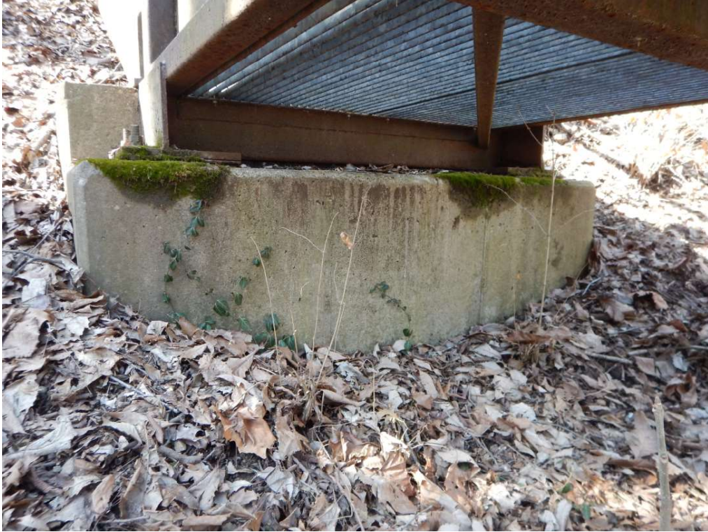
Typical Abutment Condition
