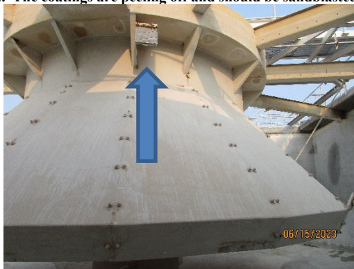
The launders are starting to rust and need to be re-coated. The coatings are peeling off and should be sandblasted and re-coated.
