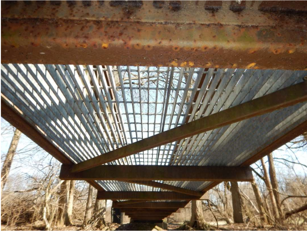
Typical Steel Underside
