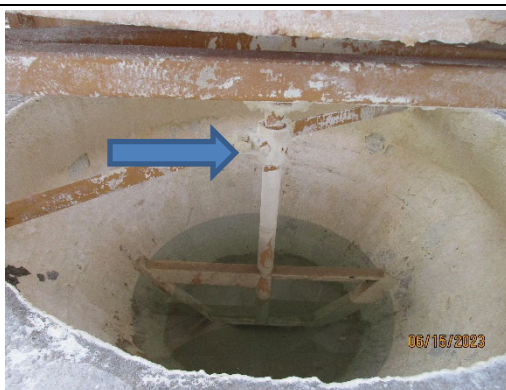
The shaft stabilizer bushing needs to be replaced.
