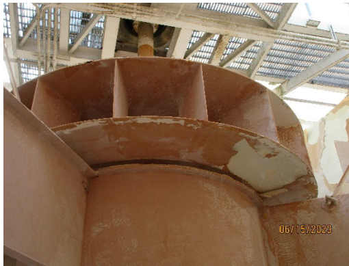
The launders are starting to rust and need to be re-coated. The coatings are peeling off and should be sandblasted and re-coated.
