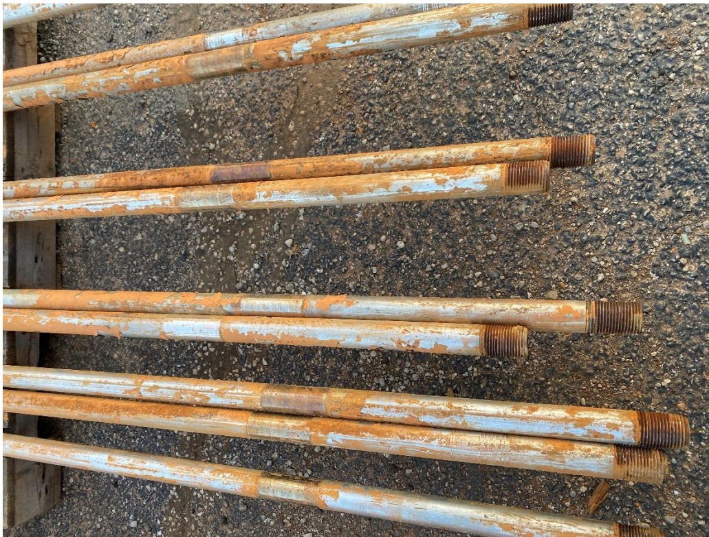
Photo 6: Close up View of Line Shafts, Signs of Wearing are Visible
