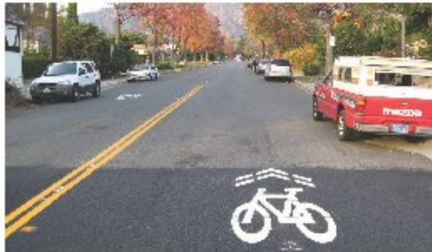
On road markings need to be clear.
