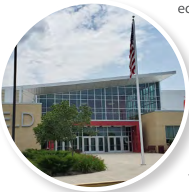
New Fairfield Freshman School constructed in 2018
