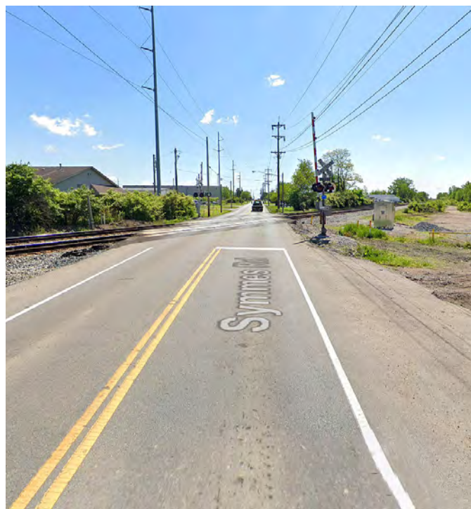
Symmes Road at CSX Rail crossing
