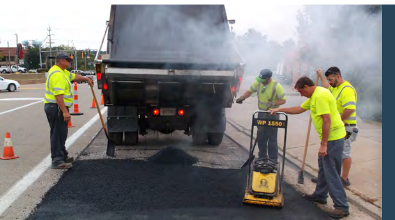
Public Works repairing city road
