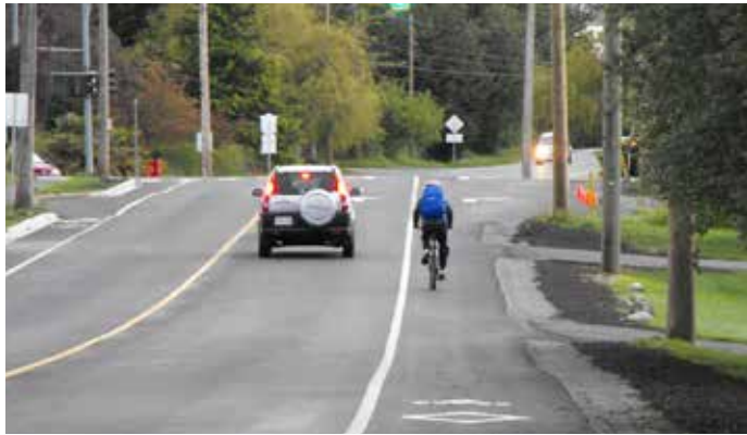
Separation of bicyclists and automobiles is crucial.
