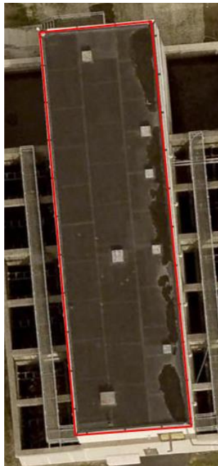
Fairfield Wastewater Filter Building
