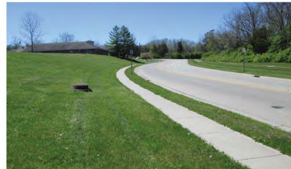
Augusta Boulevard near Pleasant Avenue.
