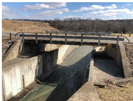
Dam Principal Spillway Photograph
