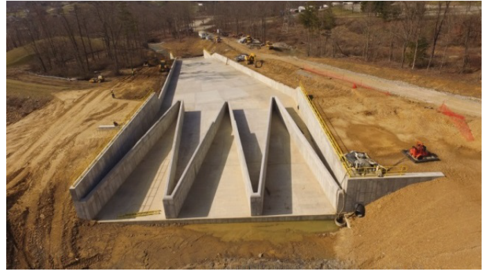
Dam No. 3 Construction
