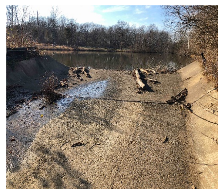
Dam Principal Spillway Photograph
