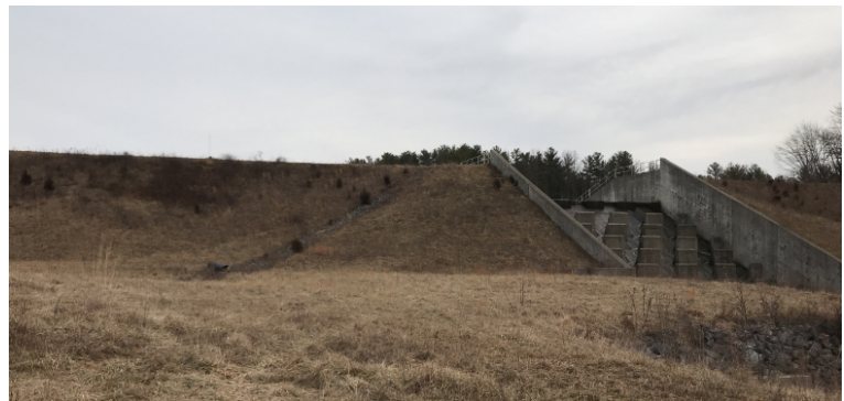
Dam Embankment and Concrete Chute Principal Spillway
