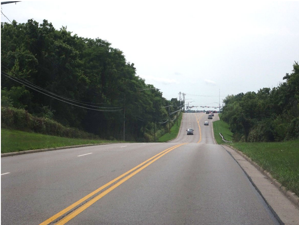
Looking south (Resor towards Mack) existing wall will be removed and poles moved back as needed. Proposed sidewalk on east side of the road between Resor and Mack.
