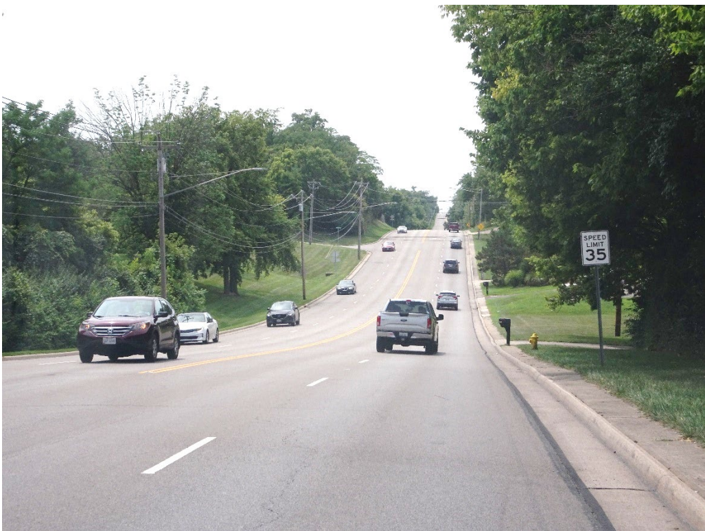
Looking south (Route 4 towards Resor) improved sidewalk up to Planet. Wide existing lanes with curb and gutter. Limited sight distance for most of S. Gilmore from Route 4 to Mack.
