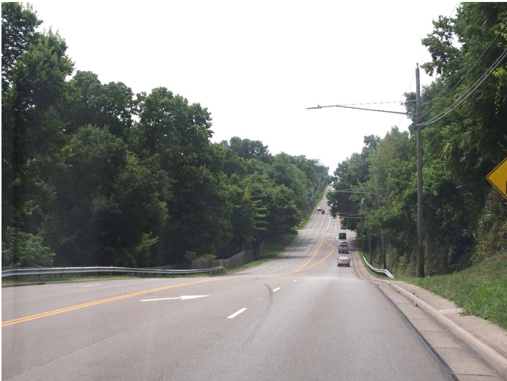
Looking south (Route 4 towards Resor) existing merge leads to congestion, ACD accidents, and aggressive driving. Trees on the west side approaching the intersection will be removed.
