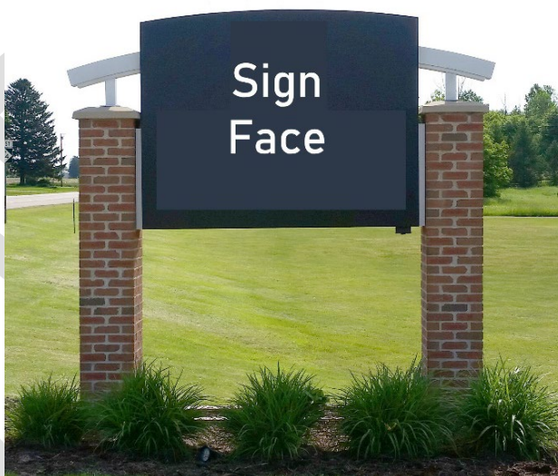
Figure 1155-6: Example of a pole sign
