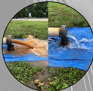
Perform Well Rehab Treatments
