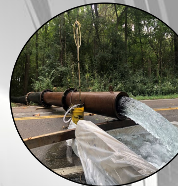
Post-Rehab Flow Test
