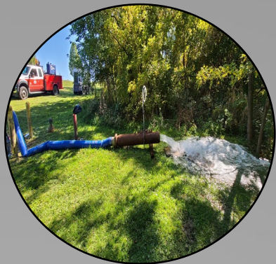
Pre-Rehab Flow Test
