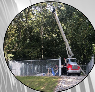
Owner's Repaired Pump Reinstalled
