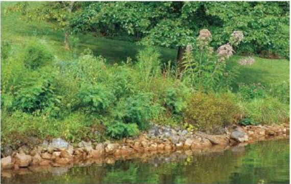
VEGETATED EDGE CONDITION
