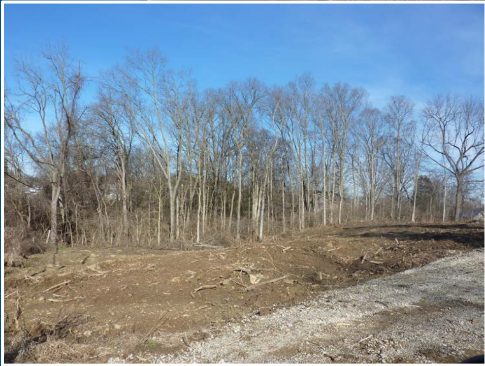
View of site looking north
