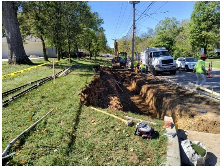
Excavation for retaining wall on Resor Road
