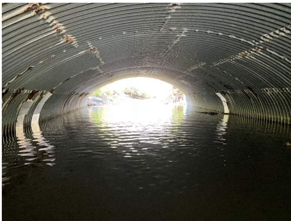
Photo 6 – Typical Underside Looking West
