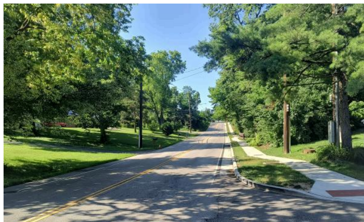
Completed sidewalk on Ross Road
