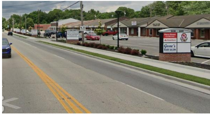
Sidewalk Improvement as part of Pleasant Avenue project
