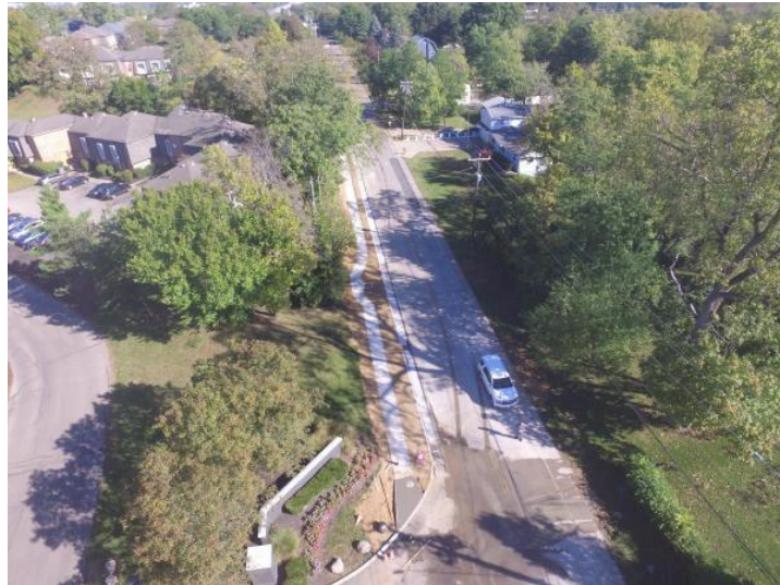
Drone photo of Ross sidewalk under construction
