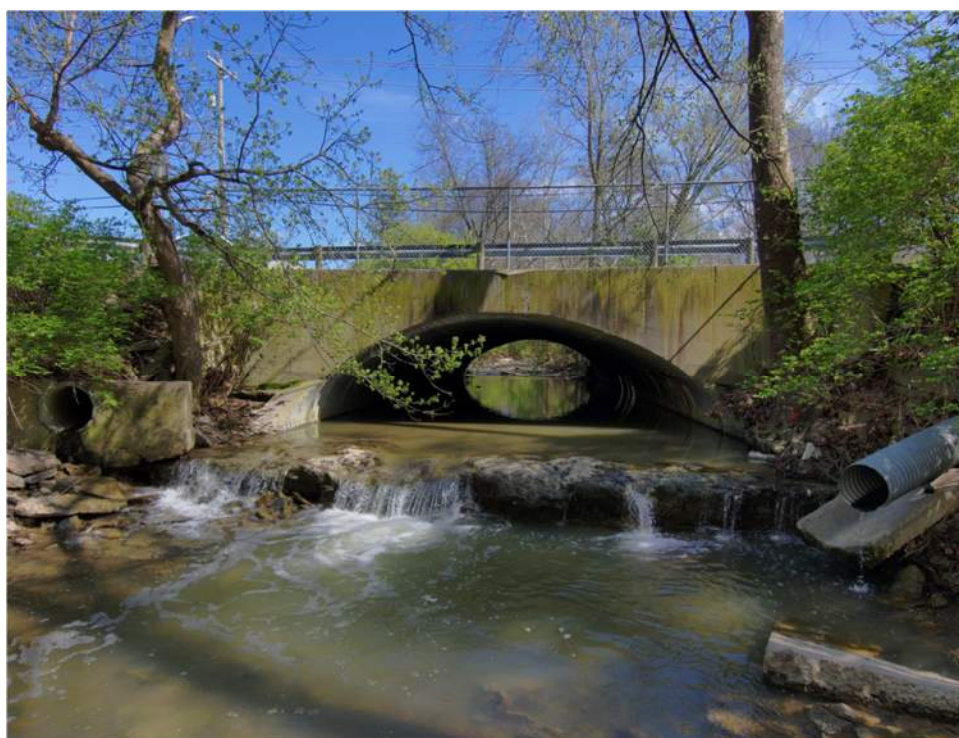
Photo 4 – West Fascia Looking East
