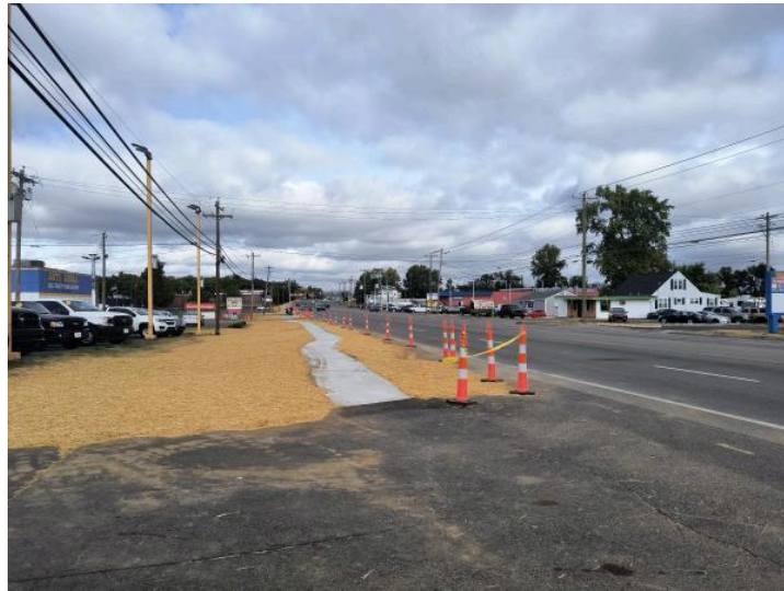
Route 4 Sidewalk between Camelot Drive and Nilles Road (west side of Route 4)
