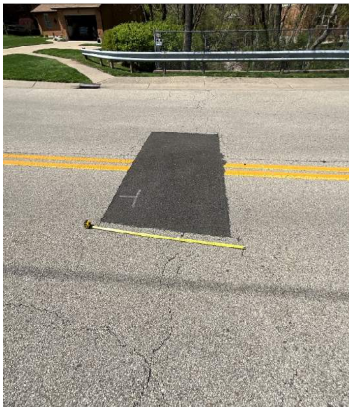
Photo 11 – Patch in Roadway Complete (2025)
