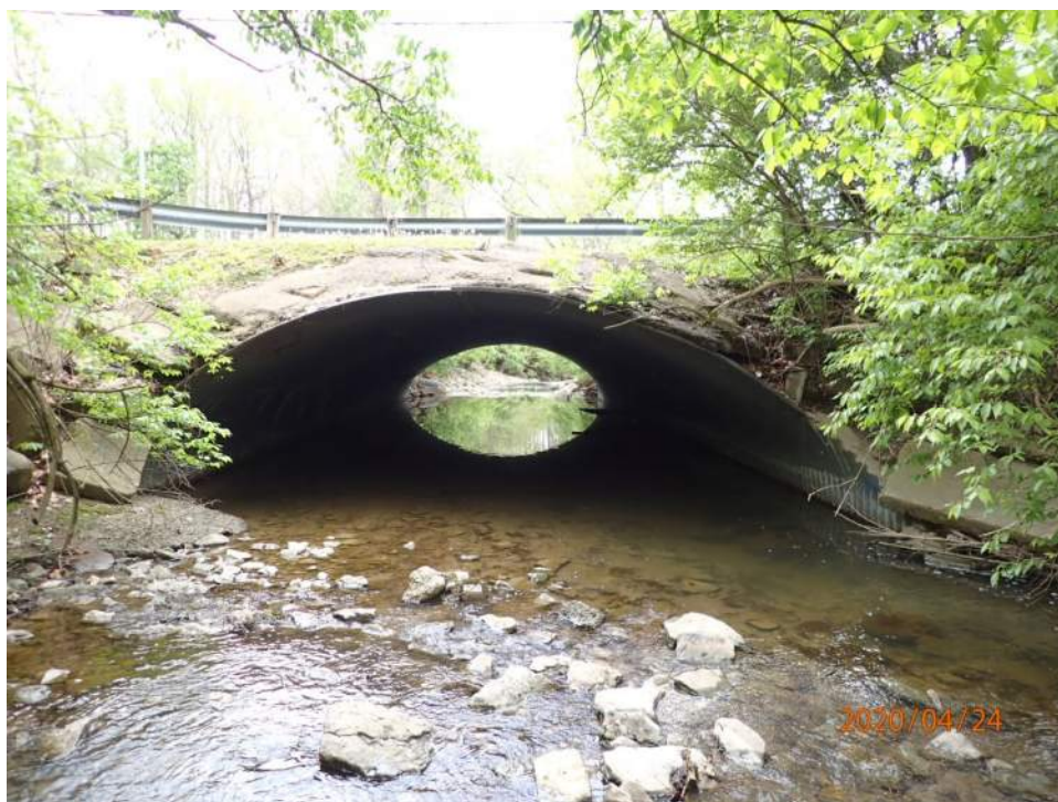
Photo 5 – East Fascia Looking West
