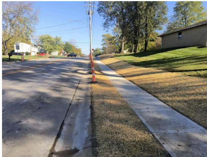
Completed Resor Road sidewalk
