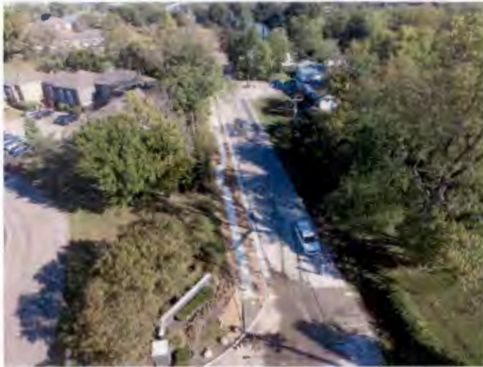
Drone photo of Ross sidewalk under construction
