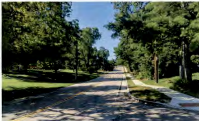
Completed sidewalk on Ross Road
