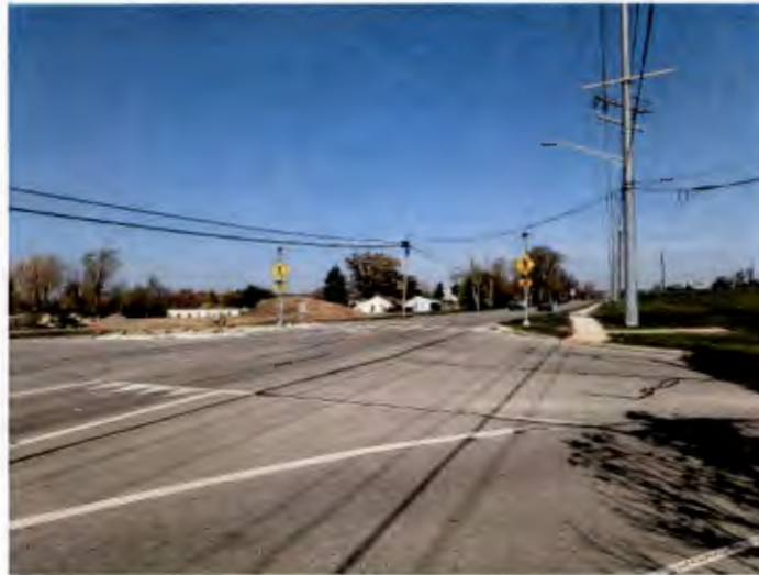
Rapid Rectangular Flashing Beacon Installation on North Gilmore Connecting Jungle Jim's shopping center to the school campus
