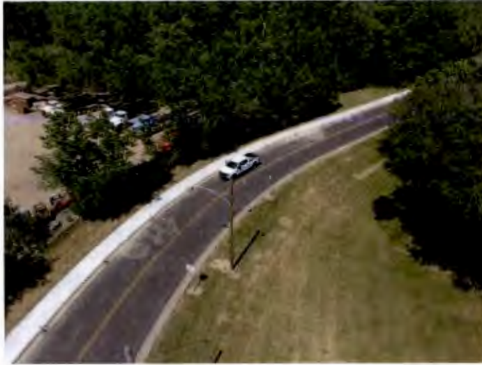
Busway Lane sidewalk construction in 2023 A second round of 2021 Funding was combined with 2022 Funding to extend the North Gilmore sidewalk and add walk along Busway and Donald
