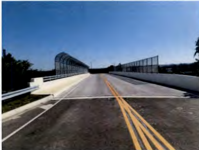
City of Hamilton Replacement of the Bilstein Bridge
