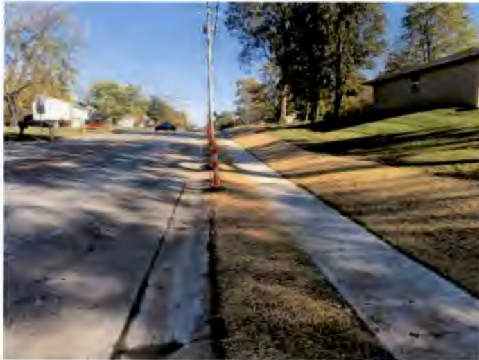
Completed Resor Road sidewalk
