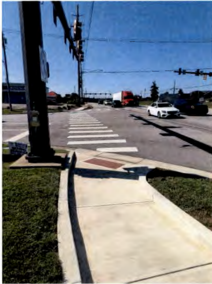
Crosswalk and Pedestrian signal installed by the City of Springdale
