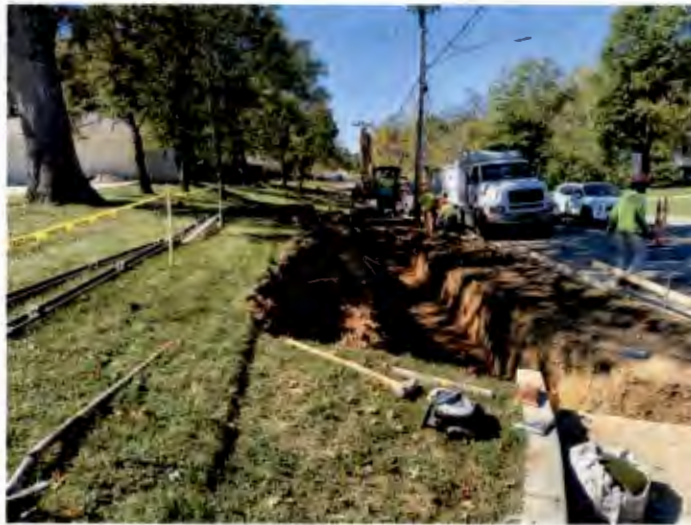
Excavation for retaining wall on Resor Road
