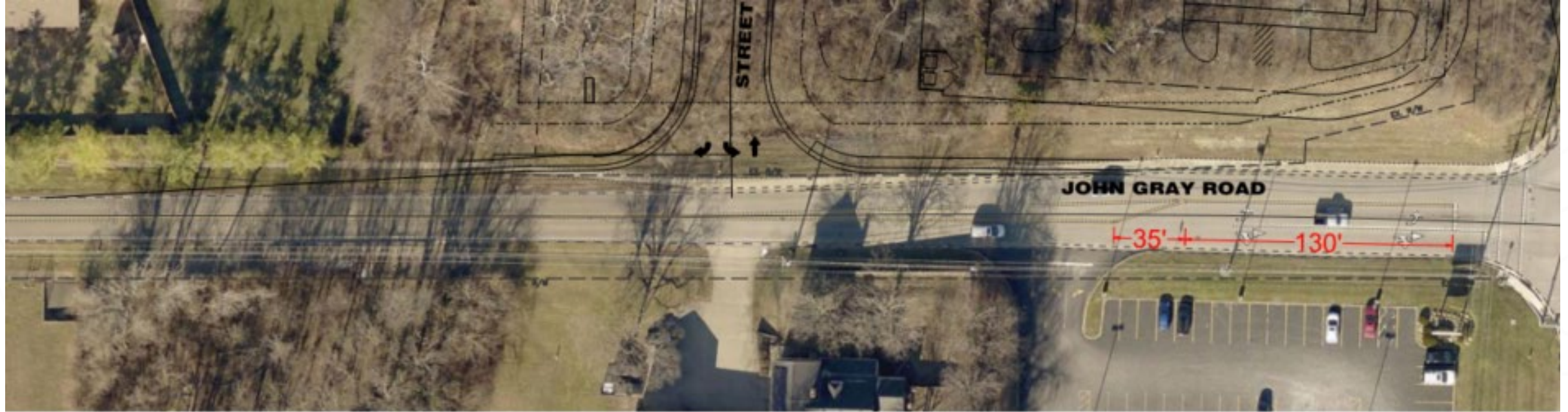
JOHN GRAY ROAD - EXISTING
