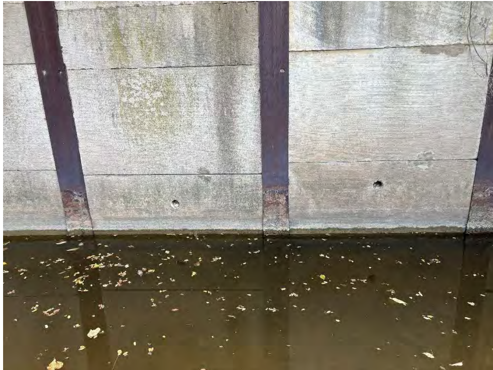
Photograph 3: Uneven weep holes due to differential downward movement of panels caused by erosion
