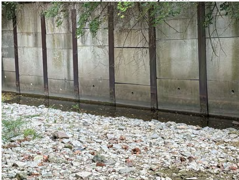
Photograph 3: Uneven weep holes due to differential downward movement of panels caused by erosion
