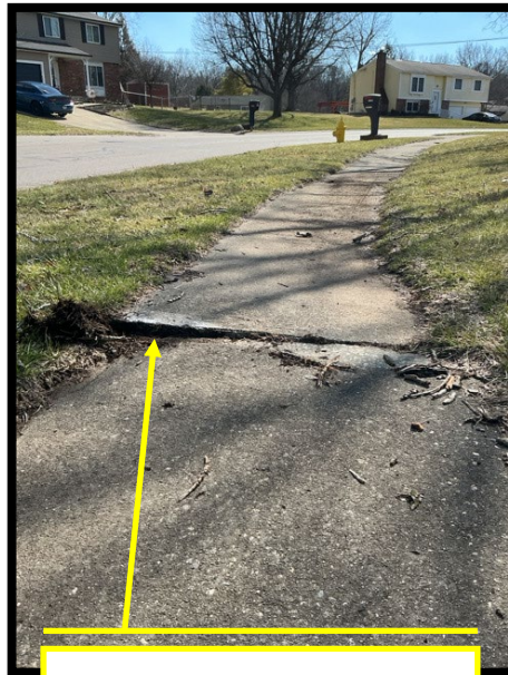
VHD 1" to 2½" TRIP AND FALL HAZARD Repairable using Precision Concrete Cutting Process
