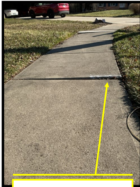
VHD 1" to 2½" TRIP AND FALL HAZARD Repairable using Precision Concrete Cutting Process
